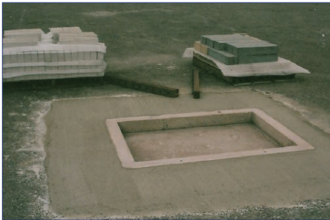
A precast slab with four-5" thick containment walls was placed in the asphalt parking lot. The paving area was 36½" x 54". The slab below the pavers was four inches thick.
